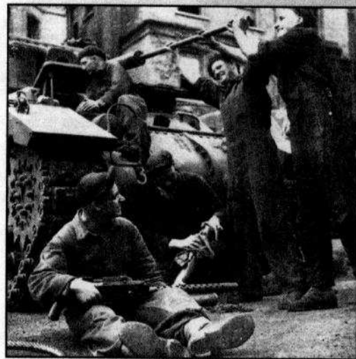
BCR Tank Maintenance
