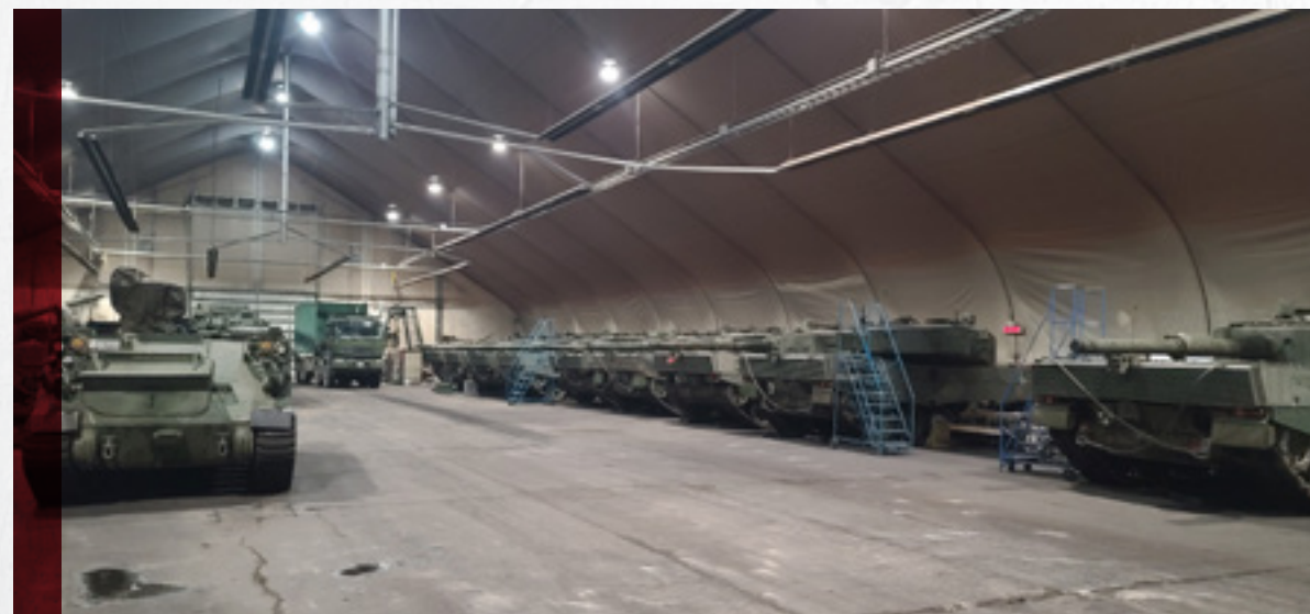
"Intended as a temporary location to store Leopard 1C2s, this decades old tent structure serves as the primary storage facility for LdSH(RC) tanks. DLI considers the temporary structure expired, and has expressed no intent to invest in its upkeep. Photo credit to Sgt Larriveé-Larouche."
